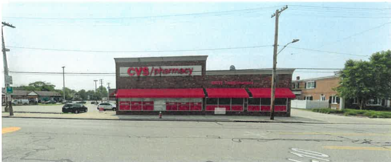
Current condition of project site (previous CVS store)
